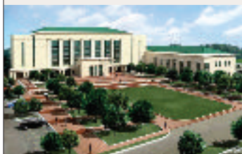
Rendering of the new Flagler County courthouse to be named after Judge Kim C. Hammond. (Courtesy of Flagler County)
